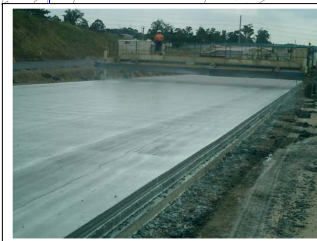
Surface Cure R being used on the M7 southwest Sydney 2005
